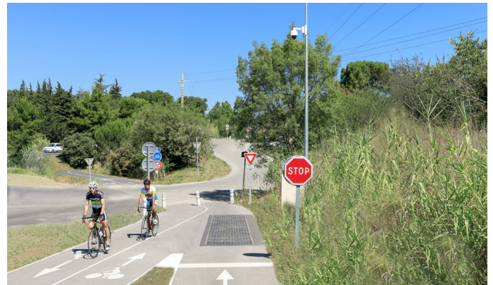
Montpellier, France - 12 panels power a CCTV camera
